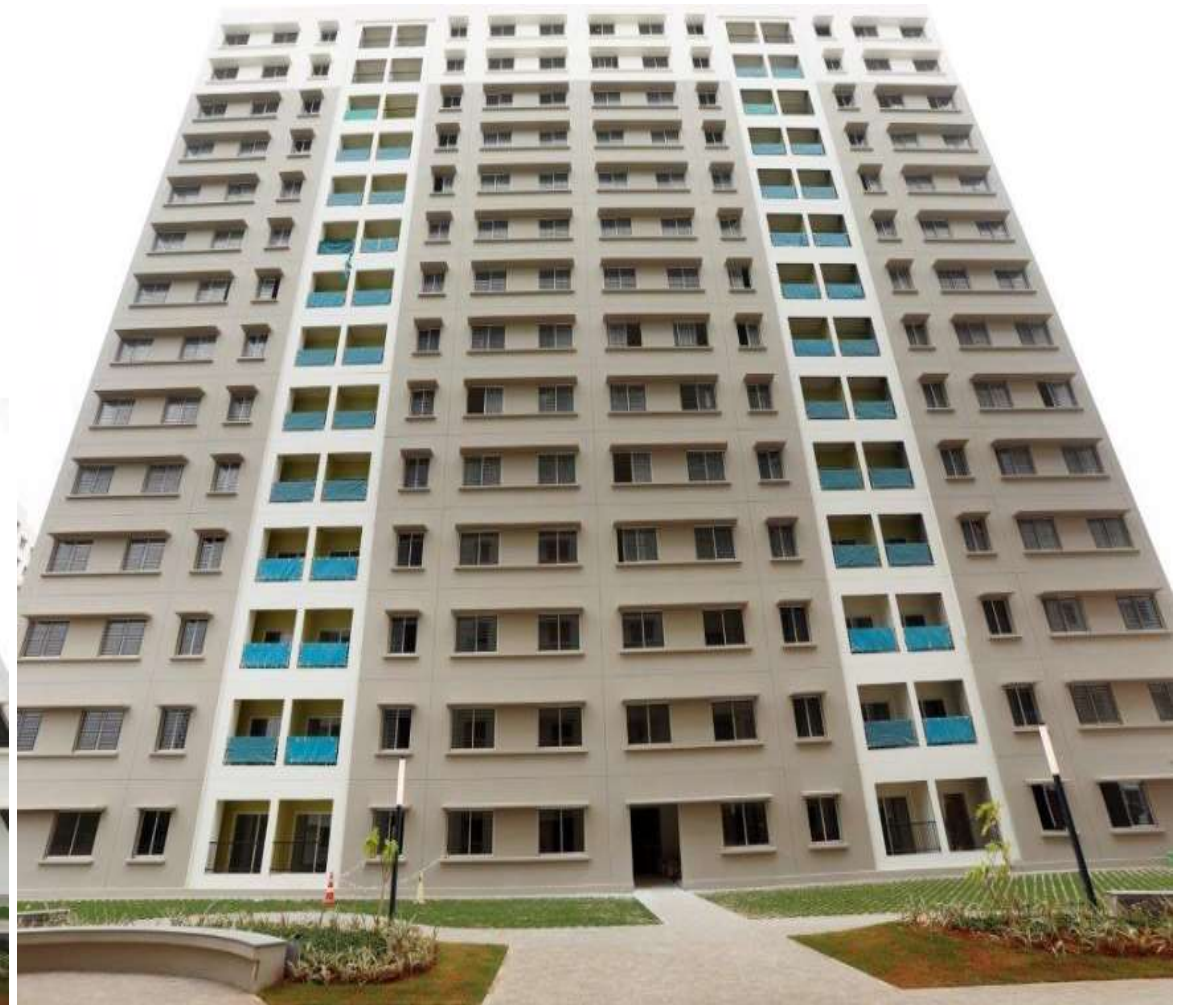
Near completion image of Wing 18 of Tropical Greens, SOBHA Dream Acres
