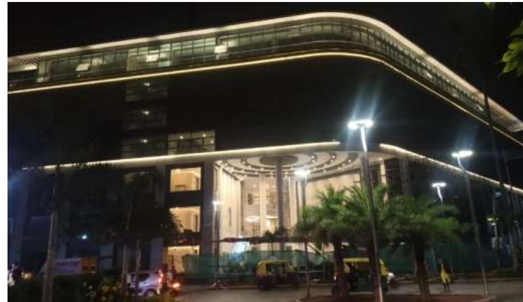
One Sobha, Bangalore- Completed
